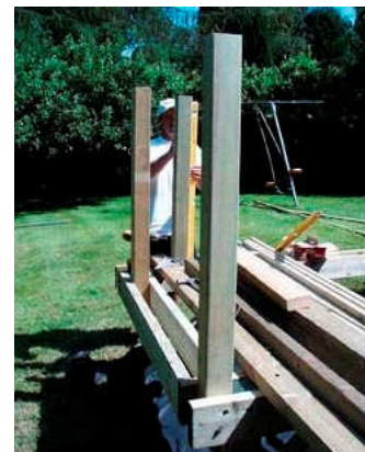
Double beams provide a ready and secure housing for balustrade newel posts
