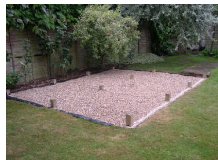
After the frame is finished and in its final position, backfill around the joists and over the weed barrier with gravel or pea shingle to a depth of 50mm.
