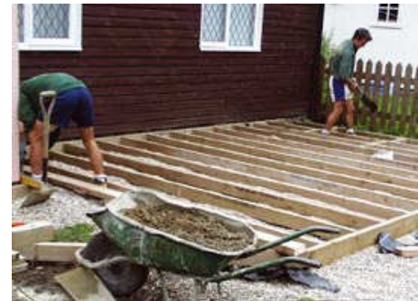
After the frame is finished and in its final position, backfill around the joists and over the weed barrier with gravel or pea shingle to a depth of 50mm.
