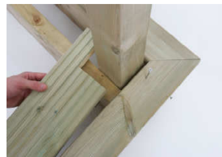
Leave a 4mm gap when fixing deck boards around newel posts to assist drainage.
